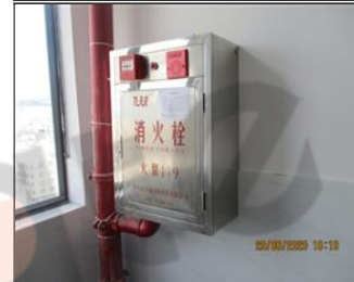
Photo of fire safety equipment Fire hydrant.JPG
