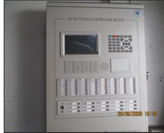
Photo of fire safety equipment Fire alarm control center.JPG
