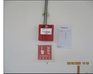
Photo of fire safety equipment Fire alarm trigger.JPG
