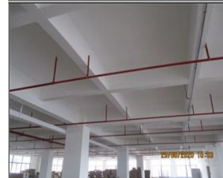
Photo of fire safety equipment Sprinkler.JPG
