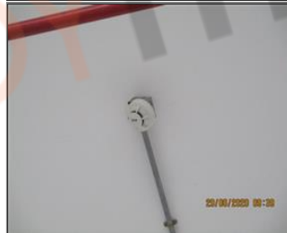
Photo of fire safety equipment Smoke detector.JPG
