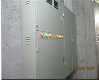
Photo of non-conformity No electric shocking warning sign posted.JPG
